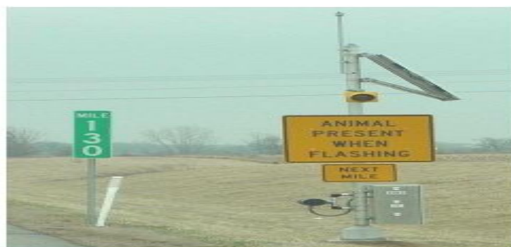
Fig. 3: The system arrangement on pole used on highway
